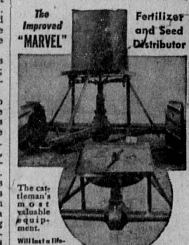
lime. FREE Folder. The above picture shows one Distributor assembled as shipped. The inset (circled) has hopper detached to show working parts and mechanism.
