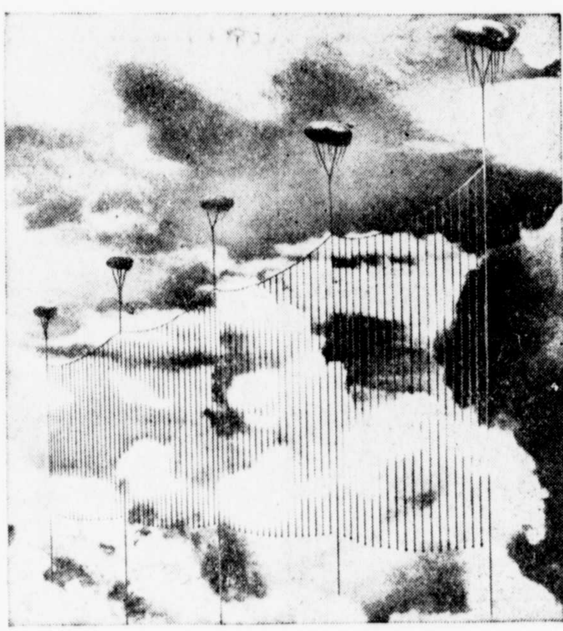
In the next war London may be defended from enemy bombers by great cable nets supported by balloons like that shown here. It is a revival of a plan of 1917 and provides a menace to low-flying planes, forcing them to fly higher, where searchlights, range finders and aircraft guns may be used against them more effectively.
