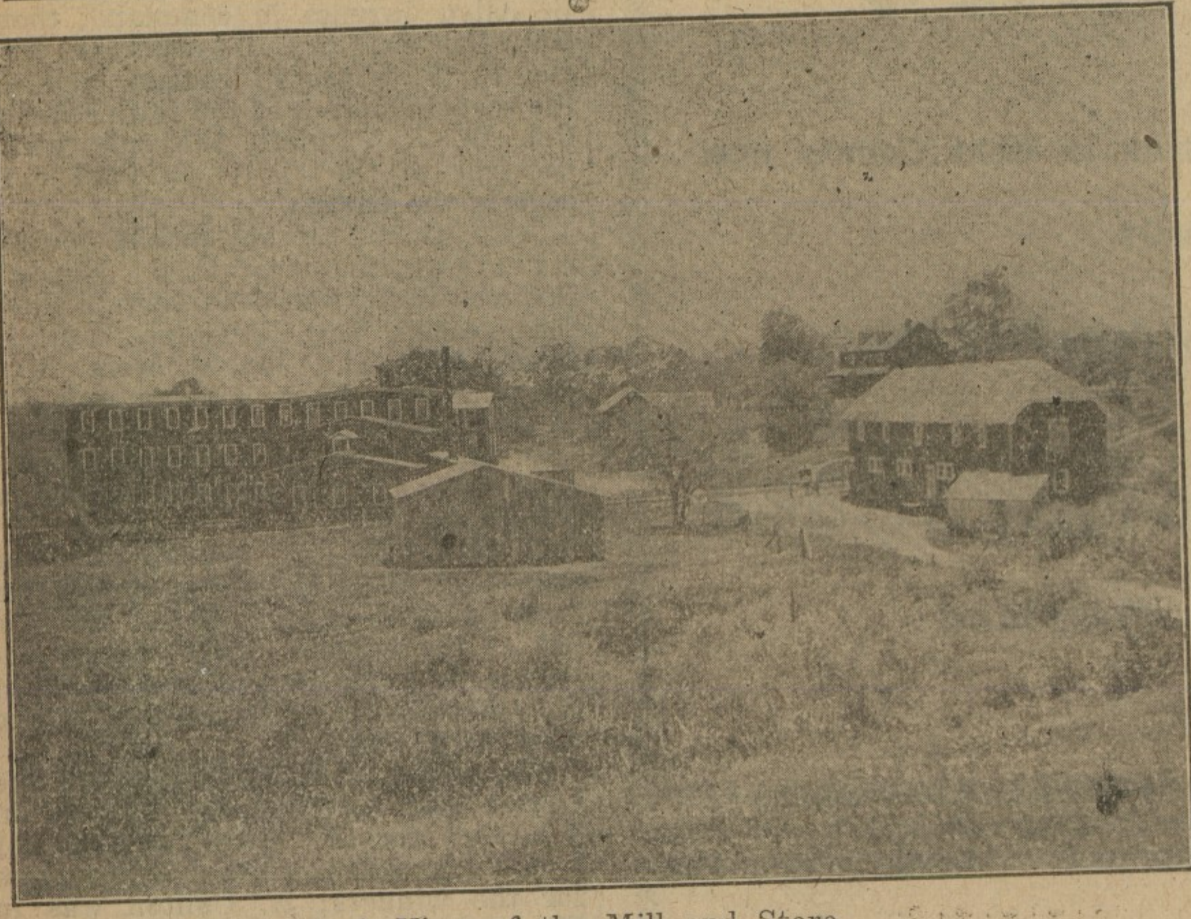
A View of the Mill and Store
